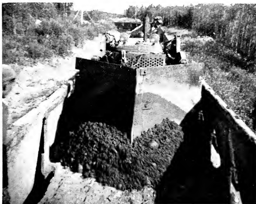
Ballast unloading plow mounted on a bulldozer.
